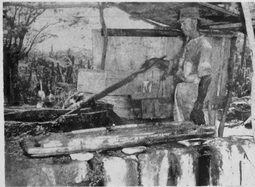
The old method of preparing aloe juice for markets needed 12 to 14 hours of boiling and stirring in copper cauldrons (see above). This made a black pitch-like substance which had to be refined in the States for aloin.
